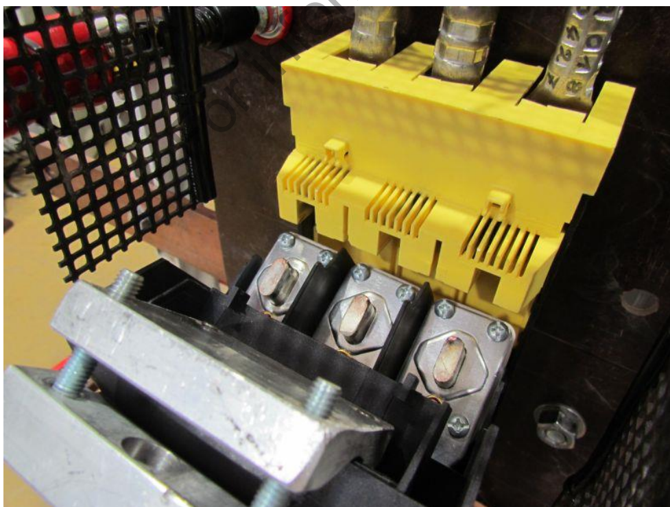
Photo 2: Test object TES-00/800 after the verification of making and breaking capacities
